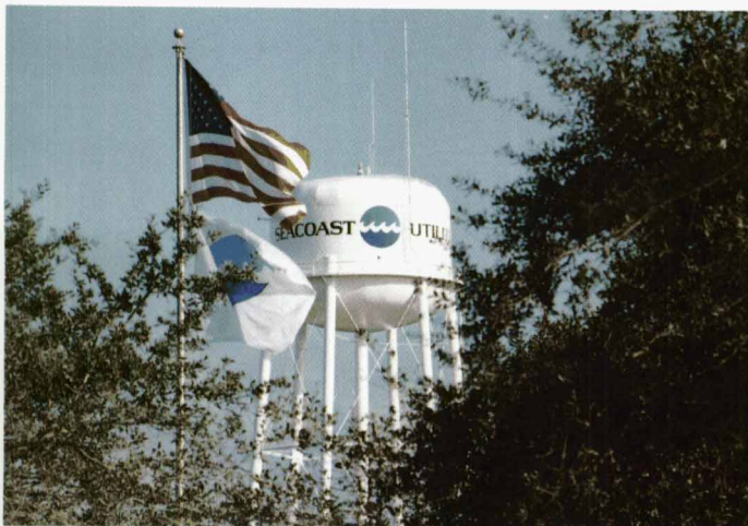
Seacoast Utility Water Tower
